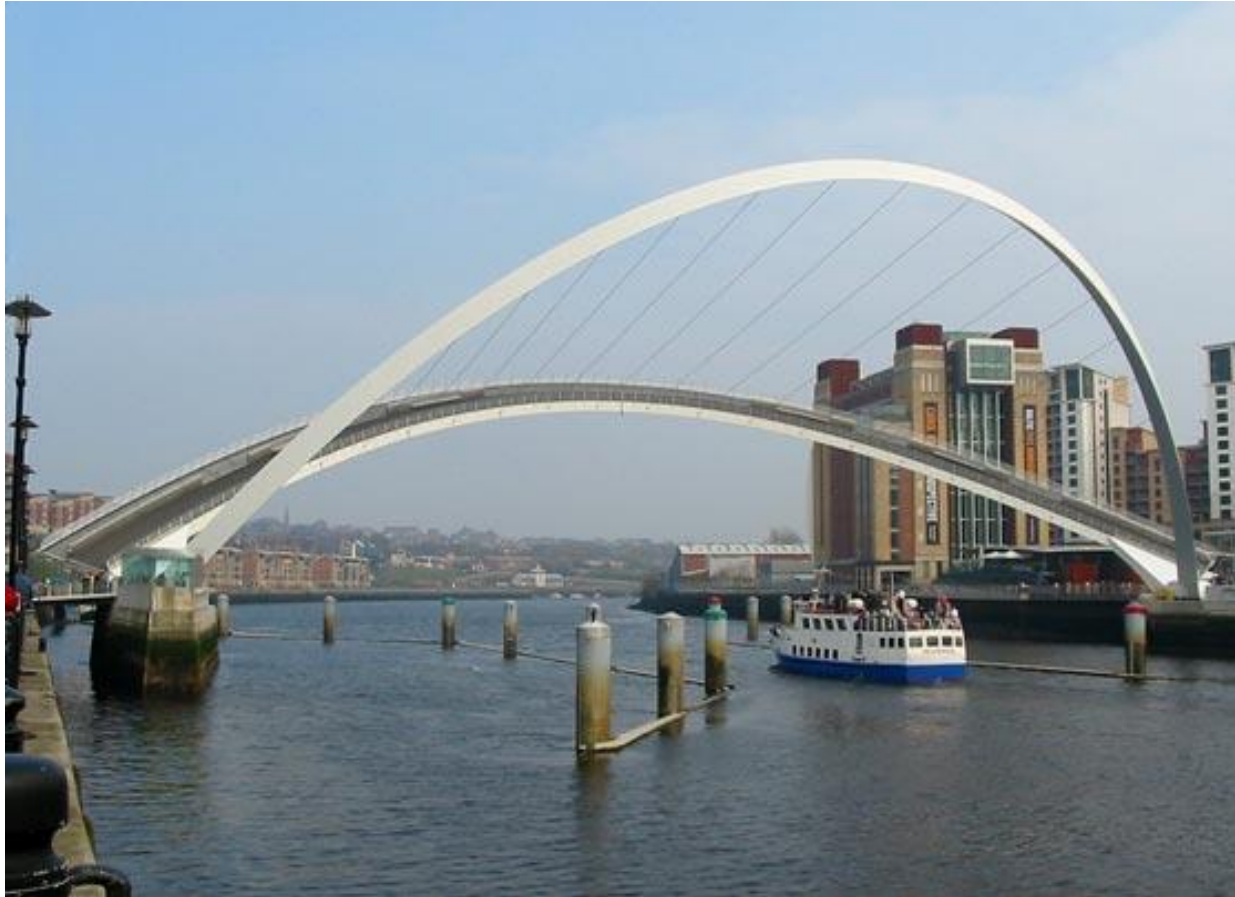
Gateshead Millennium Bridge, Newcastle, 2000
